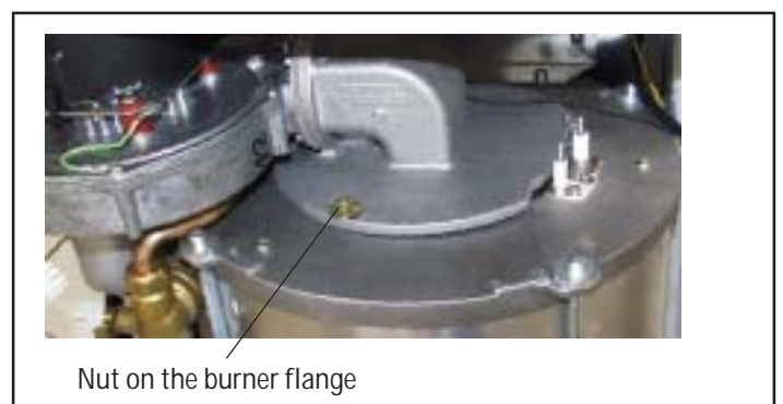
Location of nut on the burner flange
