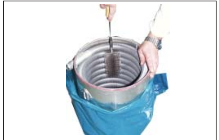
Cleaning the heat exchanger
