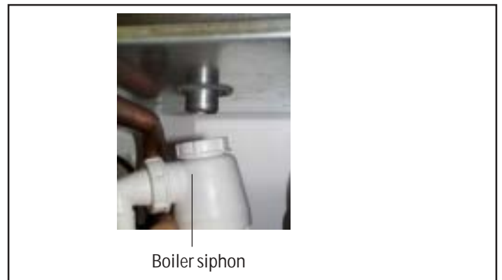
Location of boiler siphon
