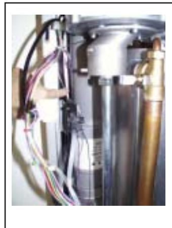
Location of boiler siphon
