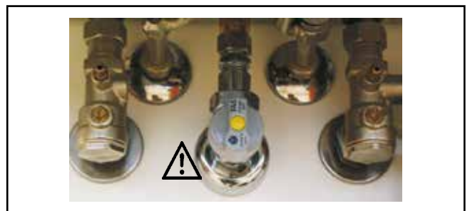
Fig.: Gas connection: Escaping gas may cause poisoning or the risk of explosion
